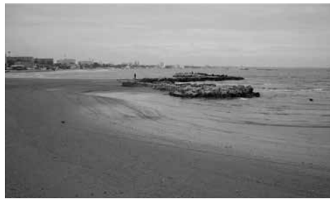
Fig. 2. Photo of coastal hydraulic structures – Mamaia breakwater
